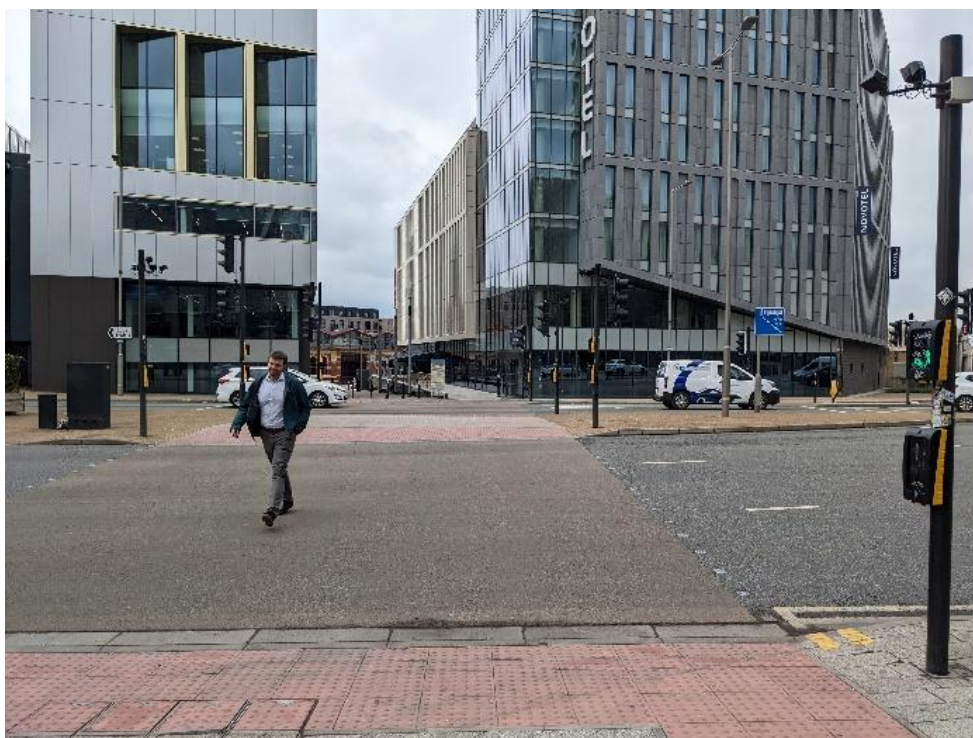
Figure 4-8 – Toucan crossing in Leicester (WSP Photograph)
