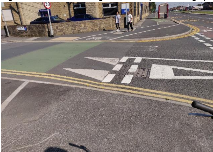
Figure 4-9 - Raised crossing in Bradford (WSP Photograph)
